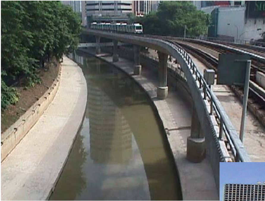
Rapid disposal approach
